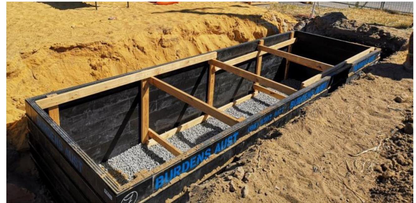
Example of bracing in a very large bespoke PLURA chamber
